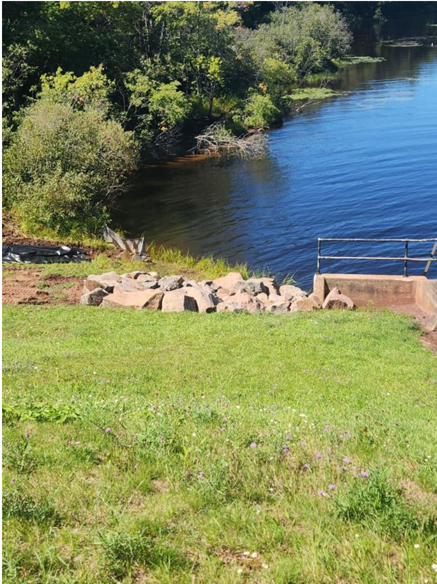
Figure 3.3.1.4-1 Completed Erosion Mitigation
