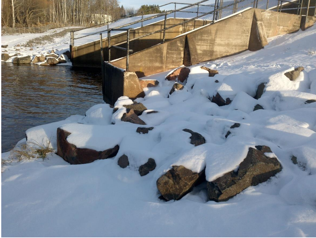
Figure 3.3.1.4-2 Completed Erosion Mitigation
