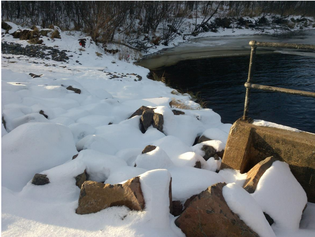
Figure 3.3.1.4-3 Completed Erosion Mitigation
